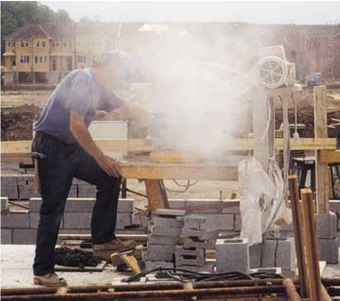
Dry cutting generates high levels of dust
